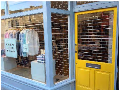
Recessed grilles behind windows.
