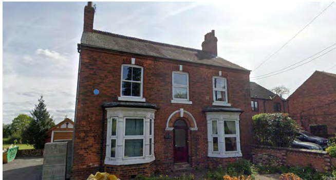
Double fronted bay windows in Ranskill.
