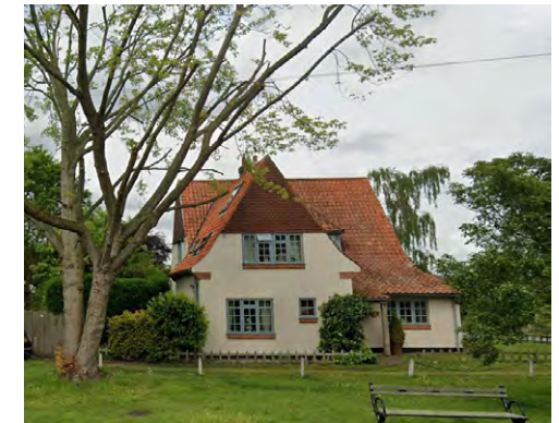
Intersecting roof gable to gable in Sutton-cum-Lound.
