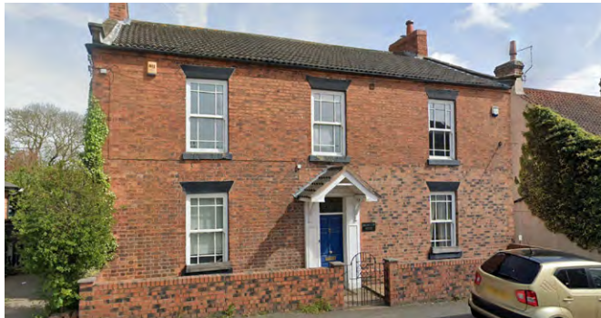
Vertically-proportioned windows on a wide elevation in Ranskill.
