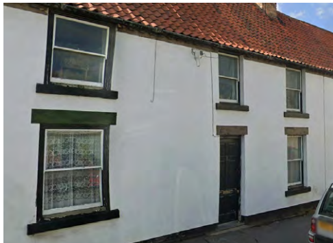
Black timber lintels and sills in Tuxford.
