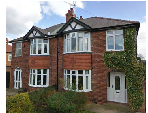
Hipped roof with slate tiles in Thrumpton.
