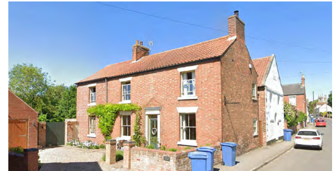
Gable end, window and door surrounds in Clayworth.
