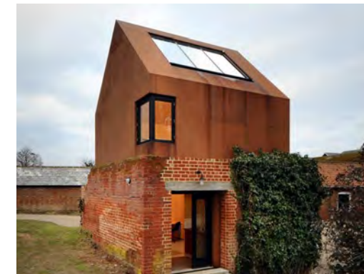
Modern cladding materials, such as Corten.
