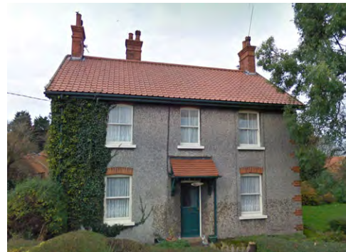
Brick chimney stacks in Scaftworth.
