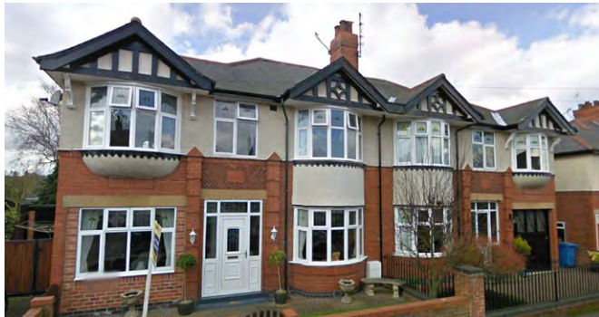
Repeated elevation features between neighbouring semi-detached houses in Thrumpton.
