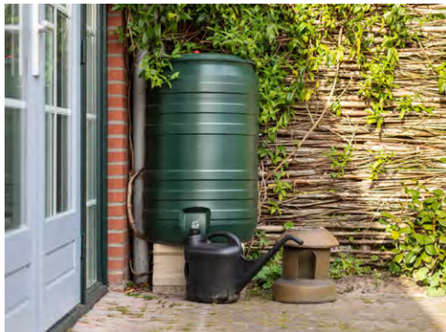
Water butts collecting water from gutters. Source: RSPB
