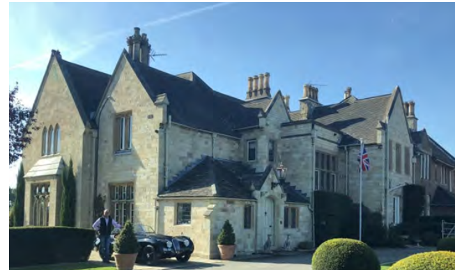
Ashlar stone at Bothamsall Hall.
