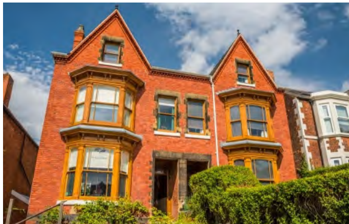
Early 20th century brickwork at Mr Straw's House, Worksop.
