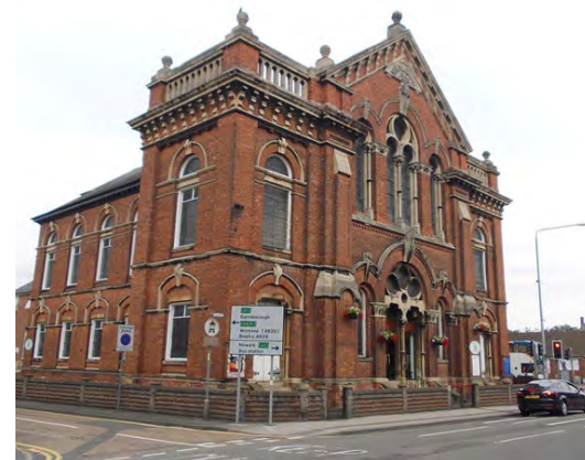
19th century brickwork at Grove St Methodist Church, Retford.
