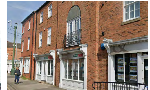
New build replicates materials, ground floor units, windows and the raised gable common on Grove Street in Retford.
