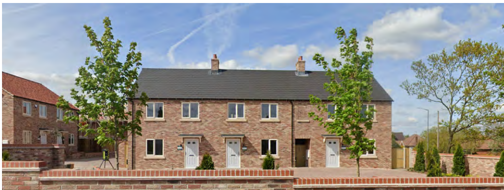
These new build homes in Ranskill pick up a variety of local street references including materials, entrances, chimney stacks, and window frames.
