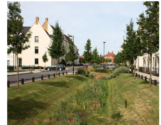
Planted strips, trenches and swales.
