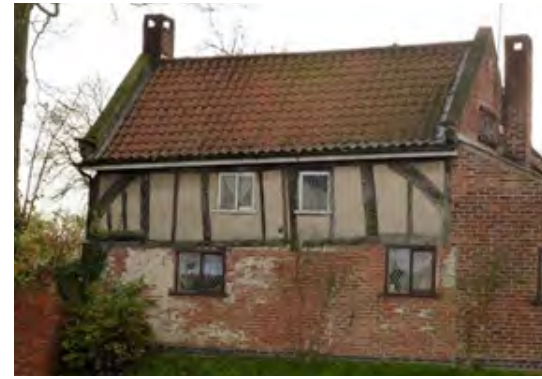
Timber framing at The Old Vicarage, Scrooby.
