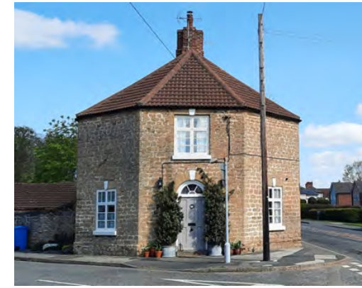
Limestone toll house at 1 High Road, Carlton in Lindrick.
