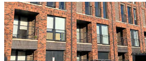
Balconies are recessed into the building elevation.
