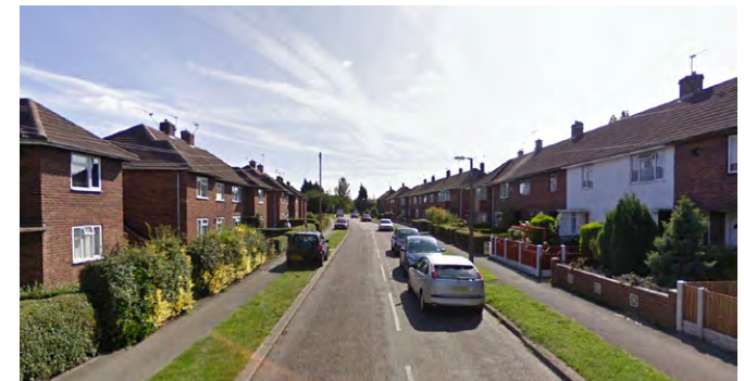
Or do all the buildings face onto the public street like in this housing area of Retford?
