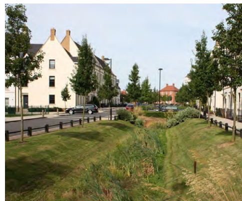
Planted strips, trenches and swales .
