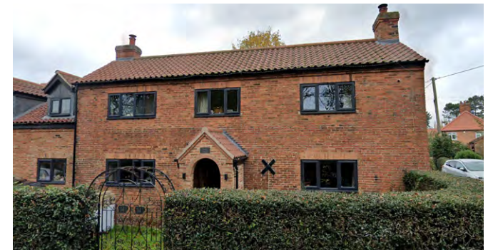
Porch details and anchor plate in Eaton.
