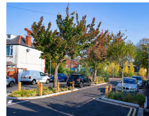
Rain gardens and bioretention tree pits in Grangetown. Source: GreenBlue Urban
